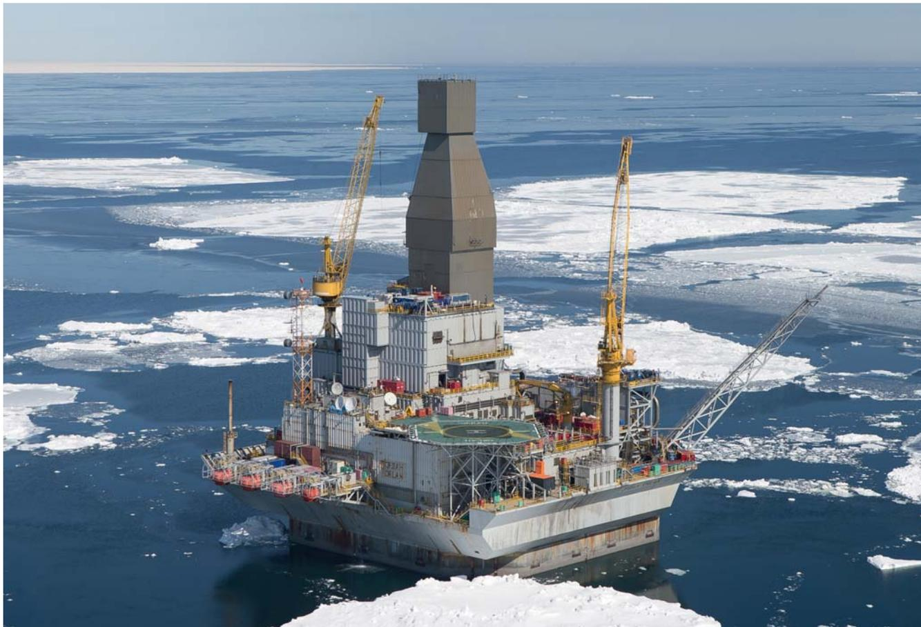
the southwestern and southeastern parts of the Chaivo field. Orlan's steel and concrete base is fit to resist ice and gigantic ice ridges rising up to a height of a six-floor house.
